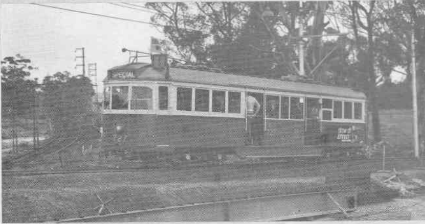
Car No.727, recently outshopped after a modification to the drop-centre is shown crossing the new bridgework in Swan St., Burnley during the T.M.S.V. tour to Carlton Control, 10th August, 1969. (Photo. Malcom Rowe)
